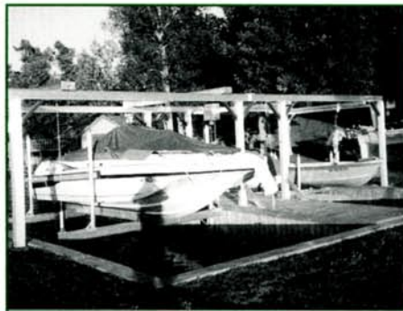
40' WIDE ALUMINUM STRUCTURE ELECTRIC REMOTE CONTROL - LIFTS 3 BOATS Pillar Point - Lake Ontario
