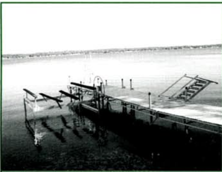
6' x 48' DOCK-HINGED TOWER 4000 LB. BOAT LIFT. 11 FEET OF WATER Point Salubrious
