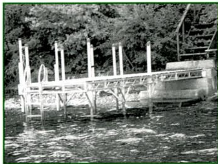
HD 6' X 32' DOCK WITH SWIM LADDER PINNED TO CONCRETE STAIRS Lake Ontario
