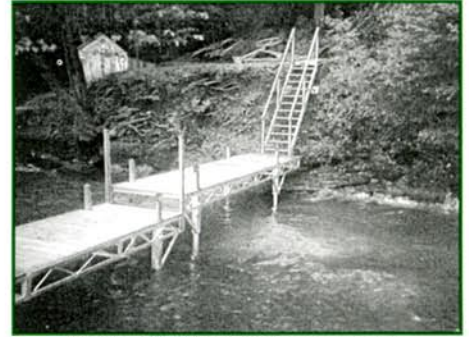
DOCK • STAIRWAY 4' X 32' WITH 6' X 16' L Otisco Lake
