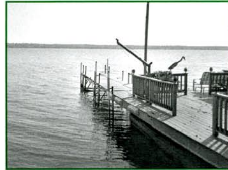
6' X 32' TOWER DOCK • HEAVY DUTY VERTICAL FENDERS • COUNTER WEIGHTED WITH SANDBAGS DOCK ACCOMMODATES 45' SEARAY LIFTS UP FOR WINTER STORAGE Pt. Salubrious - Lake Ontario
