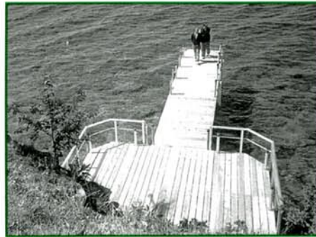
LAKE ONTARIO DOCK CABLED TO BOTTOM 12' X 16' PLATFORM WITH RAILING STEPPED DOWN TO 6' X 32' DOCK LIFTS UP FOR WINTER STORAGE
