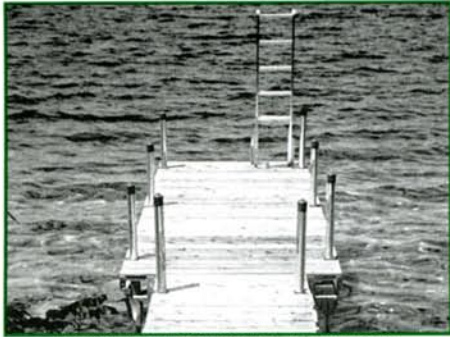
4' X 16' HINGED GANGWAY • ATTACHES TO 6'X16' HD DOCK • PINNED TO CONCRETE HD 3" ALUMINUM LEGS WITH AUGERS Lake Ontario
