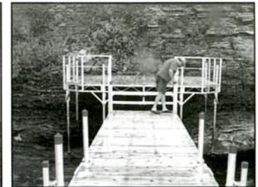
HD DOCK • 12X16 DECK STEPPED DOWN 6X32 DOCK CABLED TO ROCK BOTTOM
