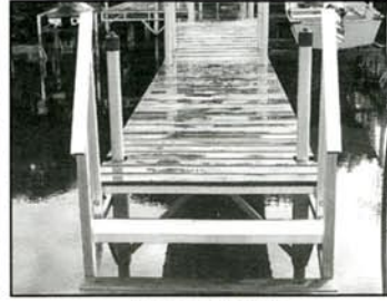
48" WIDE DOCK STEP DOWN WITH RAILINGS
